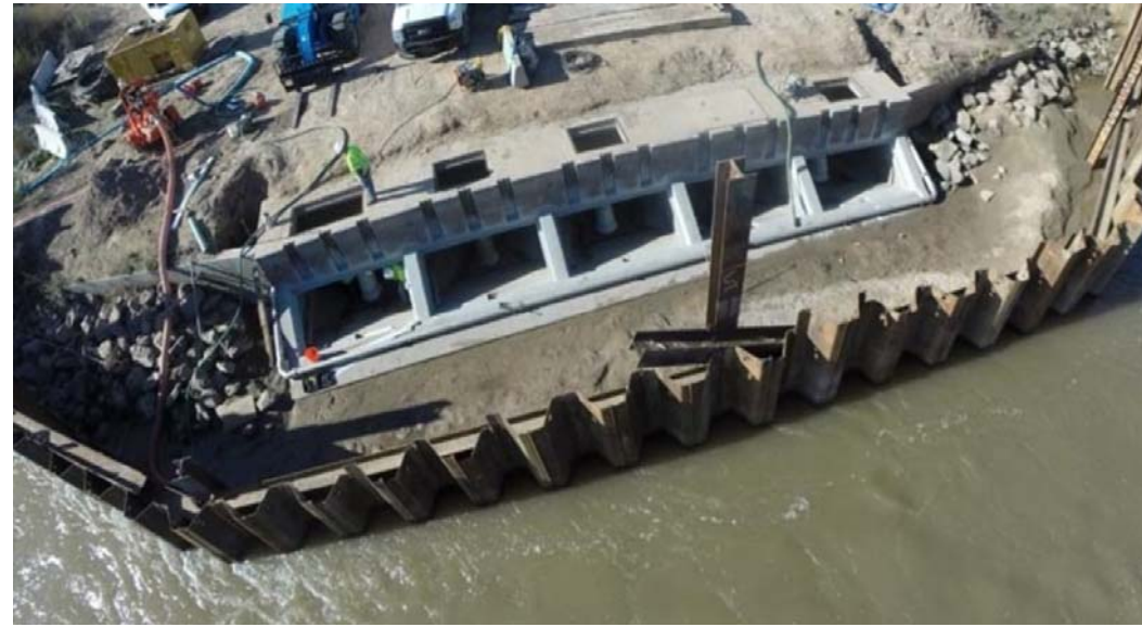
Buckman Direct Diversion Structure Under Construction
