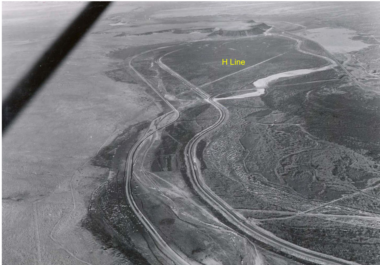
Figure 25.—Looking downstream toward San Marcial at floodway, levee, and constructed channel, December 1953 (Reclamation/Herman E. Carter). Entire flow of Rio Grande (300 cfs) is being carried by pilot channel in left of floodway. The “H Line” cut-off channel used during construction can be seen traversing the Tiffany basin.
