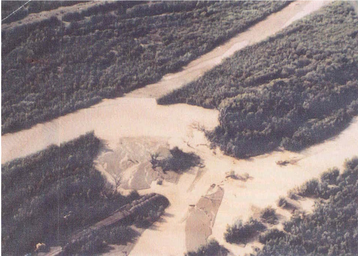
Figure 83.—Looking downstream at sediment plug and levee breach near RM 71.6 in 1991 (Reclamation/Drew Baird).
