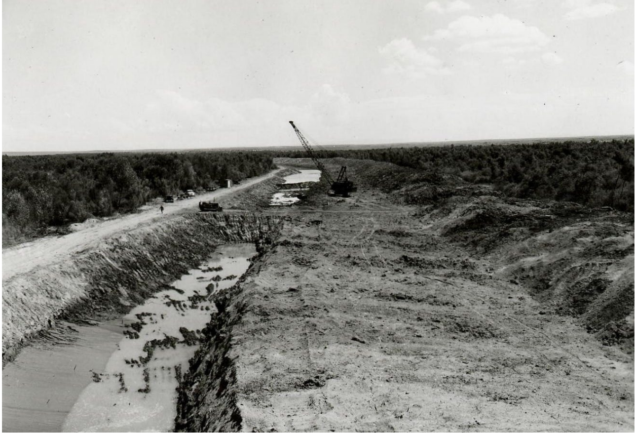
Figure 23.—Looking upstream at channel excavation operations, August 1952 (Reclamation/Herman E. Carter).
